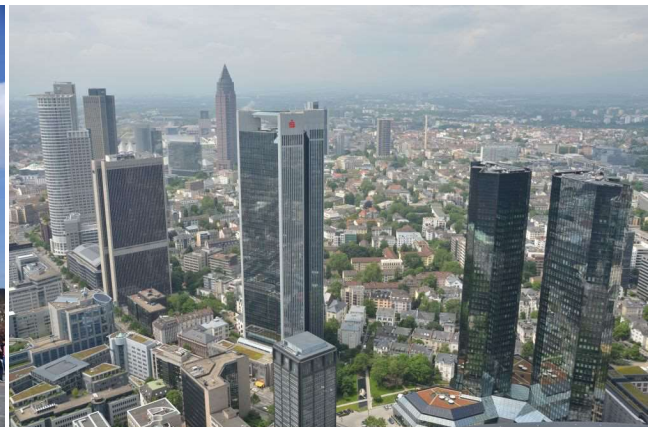
View from Maintower
